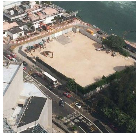
Wan Chai West Preliminary Treatment Works demolition
