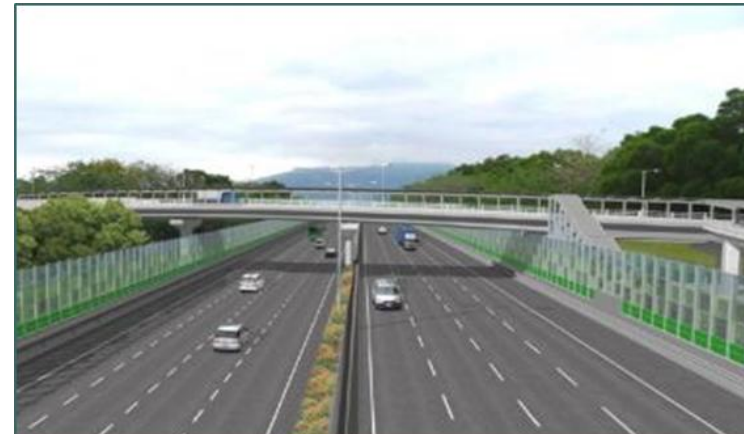
Widening of Tolo/ Fanling Highway
